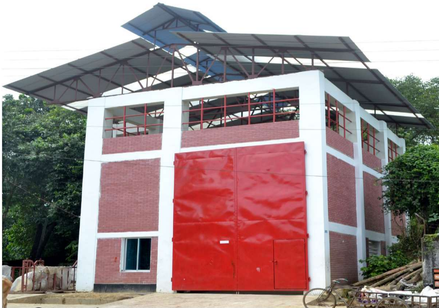
SHAHI EIDGHA-STS(secondary transfer station)
